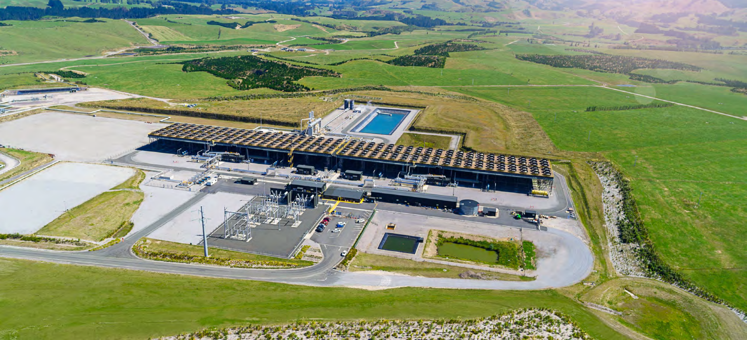
Ngā Tamariki geothermal station
