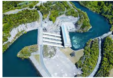
Ōhakuri (1961) 112MW 405GWh
