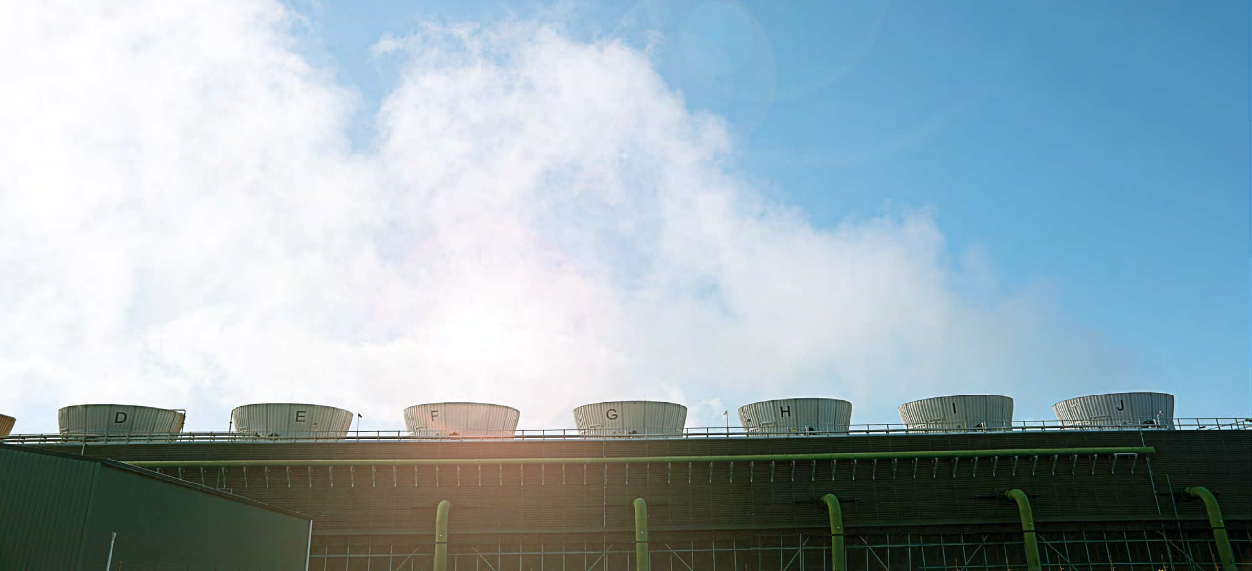
Ngā Awa Pūrua cooling tower
