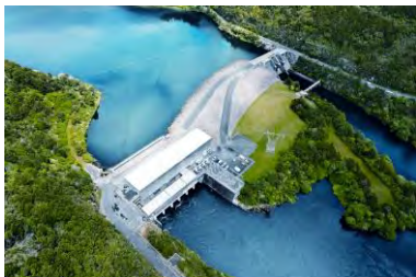
Waipāpa (1961) 51MW 235GWh
