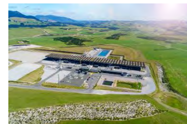
Ngā Tamariki (2013) 85MW 731GWh
