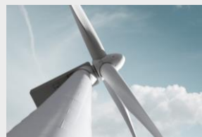
Turitea (under construction)
